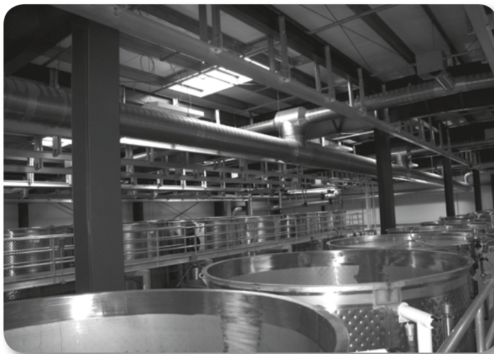
The combination of small skylights and reflection off the stainless steel equipment reduces the need for additional lighting. Also visible in the photo is the duct system.
