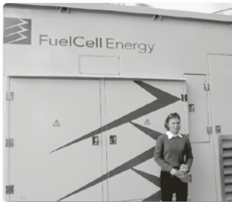
APCD Engineer Lisa Kiehl stands in front of one of two new fuel cells installed at the City of Santa Barbara's El Estero waste treatment plant. The fuel cells generate 500 kilowatts of power, providing electricity and heat for the facility's wastewater treatment system. At the same time, the system is reducing methane emissions from the plant, as the hydrogen that fuels the fuel cells is extracted from waste methane emitted by the plant.
