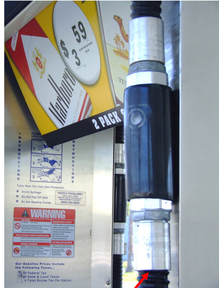
Leaking Hose Connection
