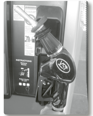
New VST (vapor systems technology) nozzles may be installed as part of the upgrade to EVR II.
