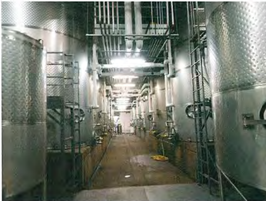
CCWS Series 400 tanks and EcoPAS piping manifold
