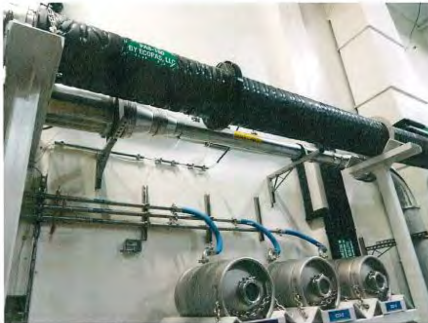
EcoPAS control system and condensate storage tanks
