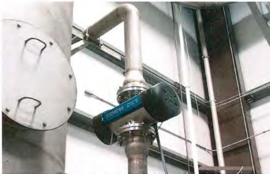
Packed bed scrubber and UV treatment lamp
