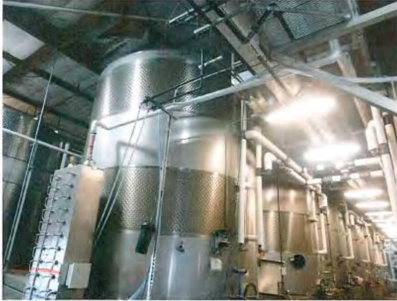
NoMoVo control system with NoMoVo piping manifold
