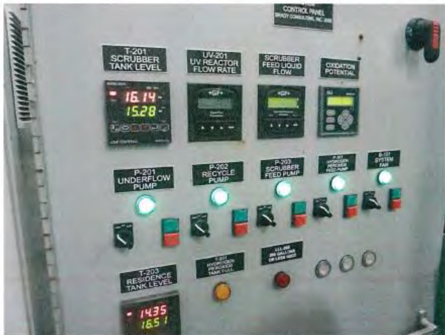
Packed bed scrubber control panel
