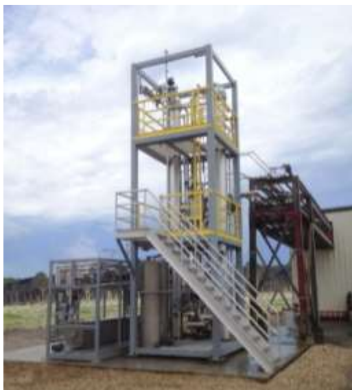
Distillation & dehydration modules installed at the University of Florida Stan Mayfield Biofuel Center
