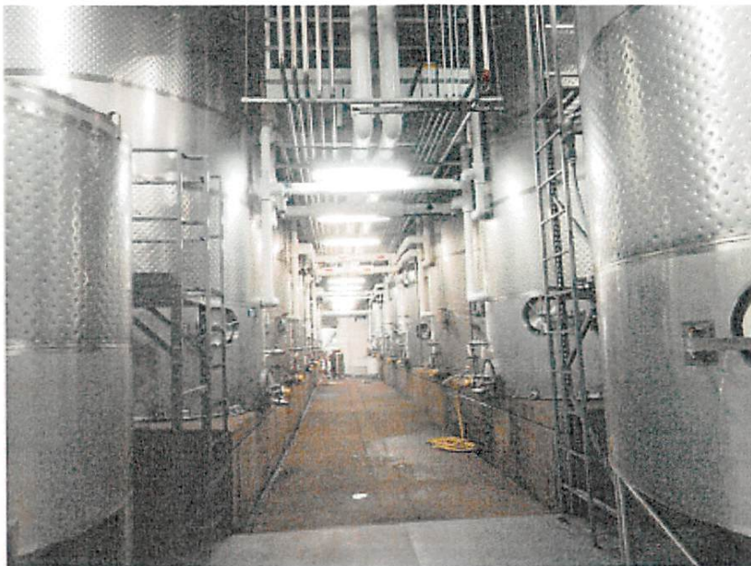
CCWS Series 400 tanks and EcoPAS piping manifold
