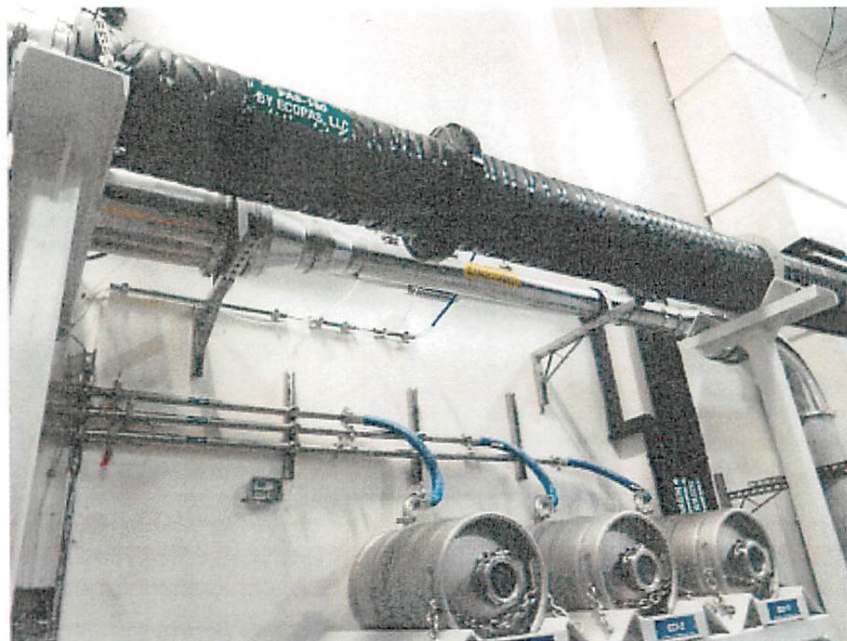
EcoPAS control system and condensate storage tanks
