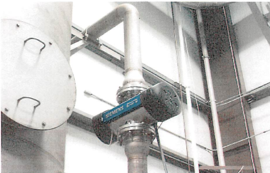
Packed bed scrubber and UV treatment lamp
