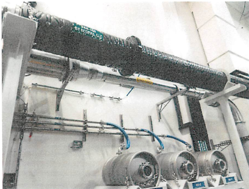
EcoPAS control system and condensate storage tanks
