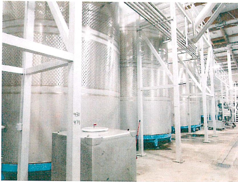
CCWS Series 400 tanks and EcoPAS piping manifold
