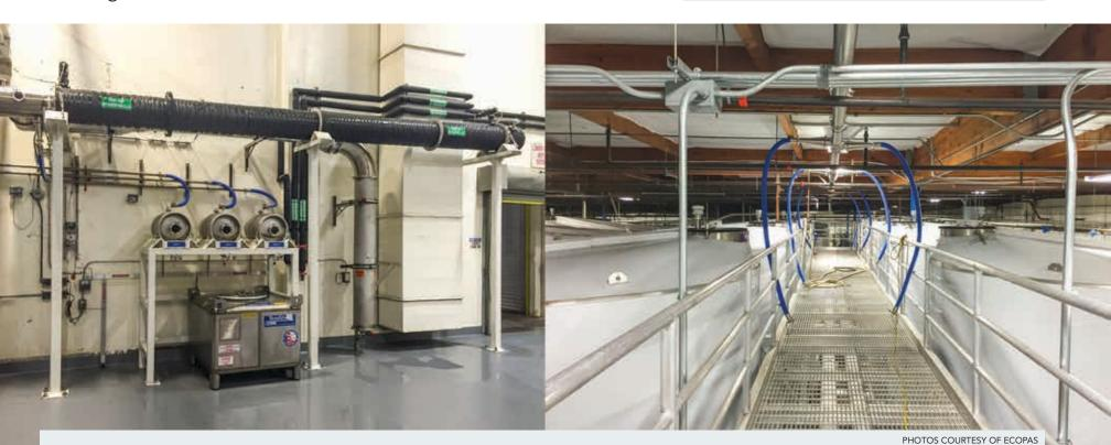
A PAS-100 unit with condenser installed at a California winery can capture volatile aroma compounds and ethanol during fermentations from multiple tanks. Blue manifold connections above a tank row catwalk can be attached to closed tank fermentors to capture volatile aromas and ethanol during fermentations using a PAS-100 unit located on the winery floor.
