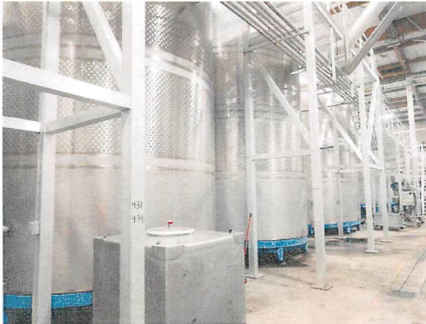
CCWS Series 400 tanks and EcoPAS piping manifold
